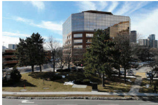
2005 Sheppard Avenue East
