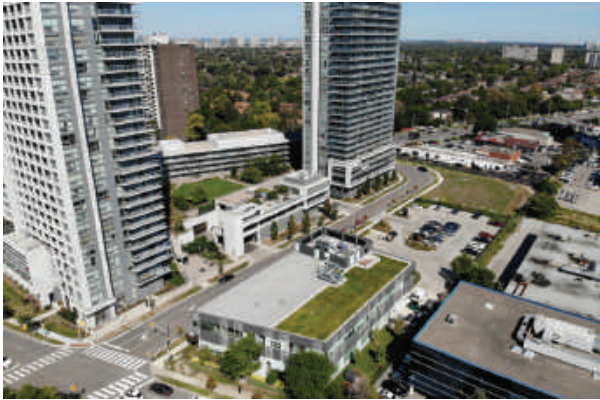
1 Heron's Hill Way- looking northeast from Yorkland Road
