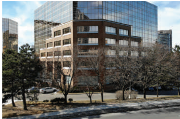
2001 Sheppard Avenue East
