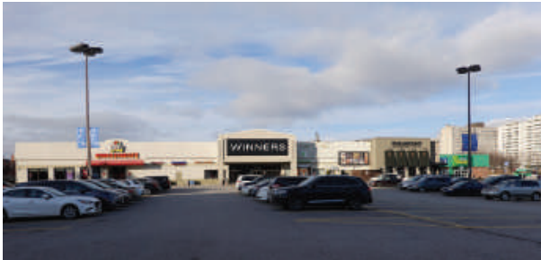
2450-2452 Sheppard Avenue East
