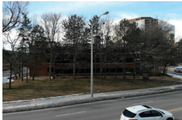
2005 Sheppard Avenue East, 3-storey parking structure
