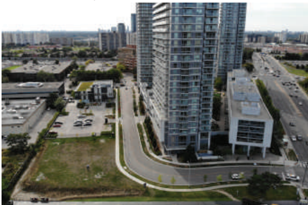
1 Heron's Hill Way- looking west
