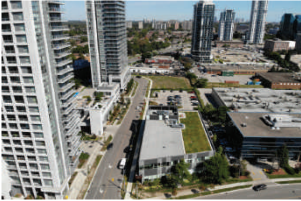
1 Heron's Hill Way- looking east from Yorkland Road
