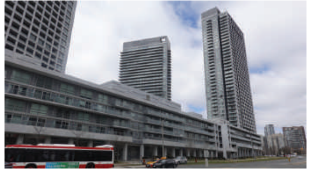
2015-2035 Sheppard Avenue East
