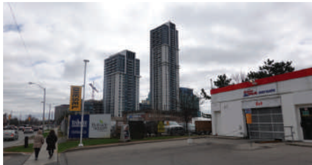
2205 Sheppard Avenue East
