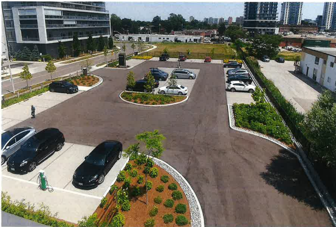
General view of parking lot and landscaped area (looking east)
