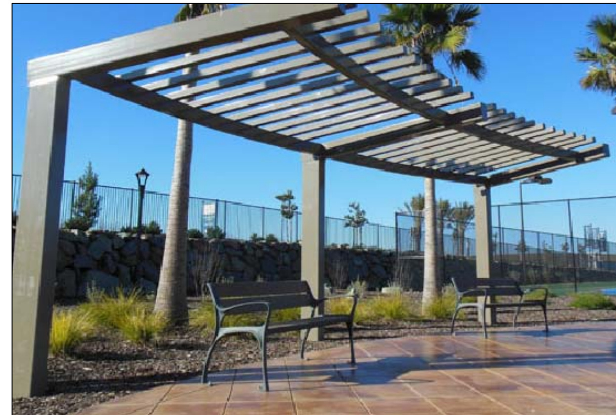
SHADE STRUCTURE (POPS)
